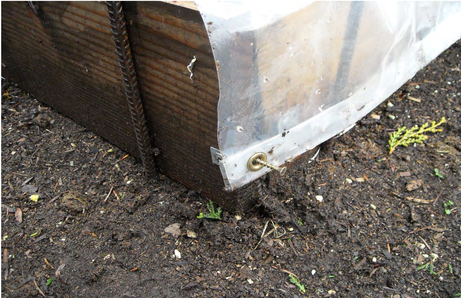
Greenhouse film doubled at the base with grommets inserted every 2-3 feet, and screwed into the board.
